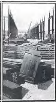
Redi-Cut System of Construction.
