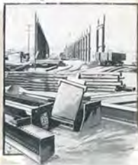
Redi-Cut System of Construction
