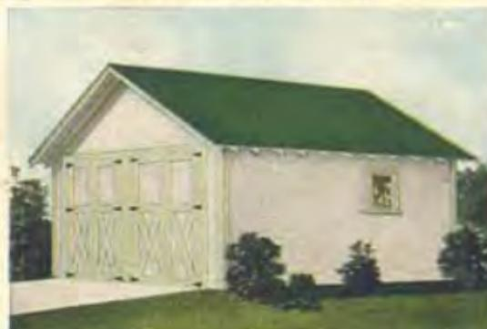
Sills 4x4 in.; studding, 2x4 in. 24-inch centers; drop siding for side walls; rafters, 2x4 in. 24-inch on centers; roof, one-quarter pitch; exposed eaves, one foot projection. Roof sheathing, laid tight. Best quality green slate surfaced roofing for roof. Garage doors furnished knocked
