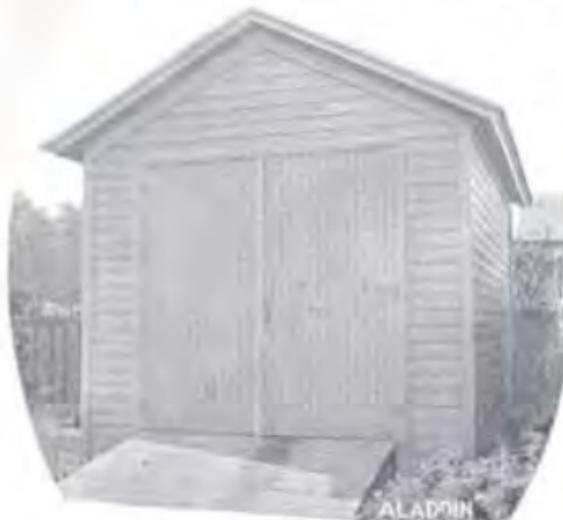
ends; joists, studding and rafters placed every 16 inches; flooring 1-inch matched; siding ½-inch tongued and grooved; roof tongued and grooved matched lumber; size of large door 8x8 feet; runway 2-inch planks. Price includes all lumber cut to fit, all hardware, locks, nails, hangers, paint, any color, for two coats. Price, complete.....\$89
