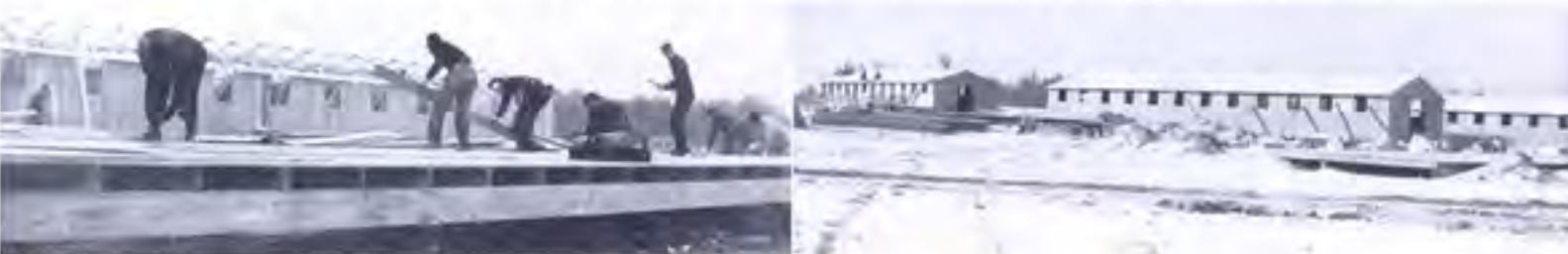
Fort Brady—Barracks and Service Buildings—Completed 10 Days Ahead of Time
