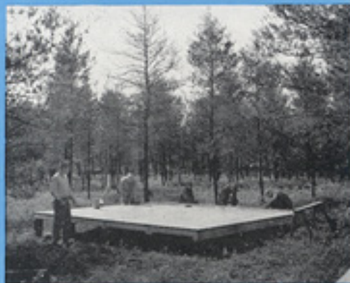
First step, laying floor section.
