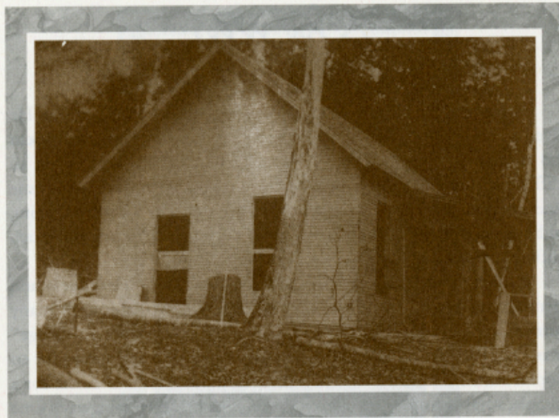
Windemere under construction.
