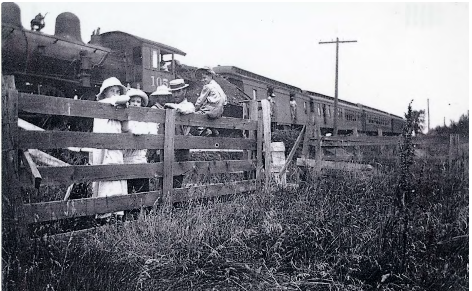
Photo #2: Next the photographer moved into the lane pictured in photo one. A lady and her parasol can be seen along the right margin. The "shot gun" stack on the engine is typical of the Pittsburgh Locomotive works "ten wheeler engine". Notice the derailed tender tilted to the east and reflecting the overcast sun of late morning.
