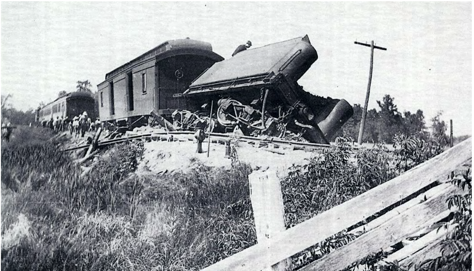
Photo #8: With the locomotive separated from the tender the former has been moved away, perhaps to the nearest siding at Forest Hill a few miles south. Torn up tracks and several large jacks are near the tender. The mail car has been put back on the track and is connected to the passenger cars in the background. A section crew can be seen repairing the right of way.
