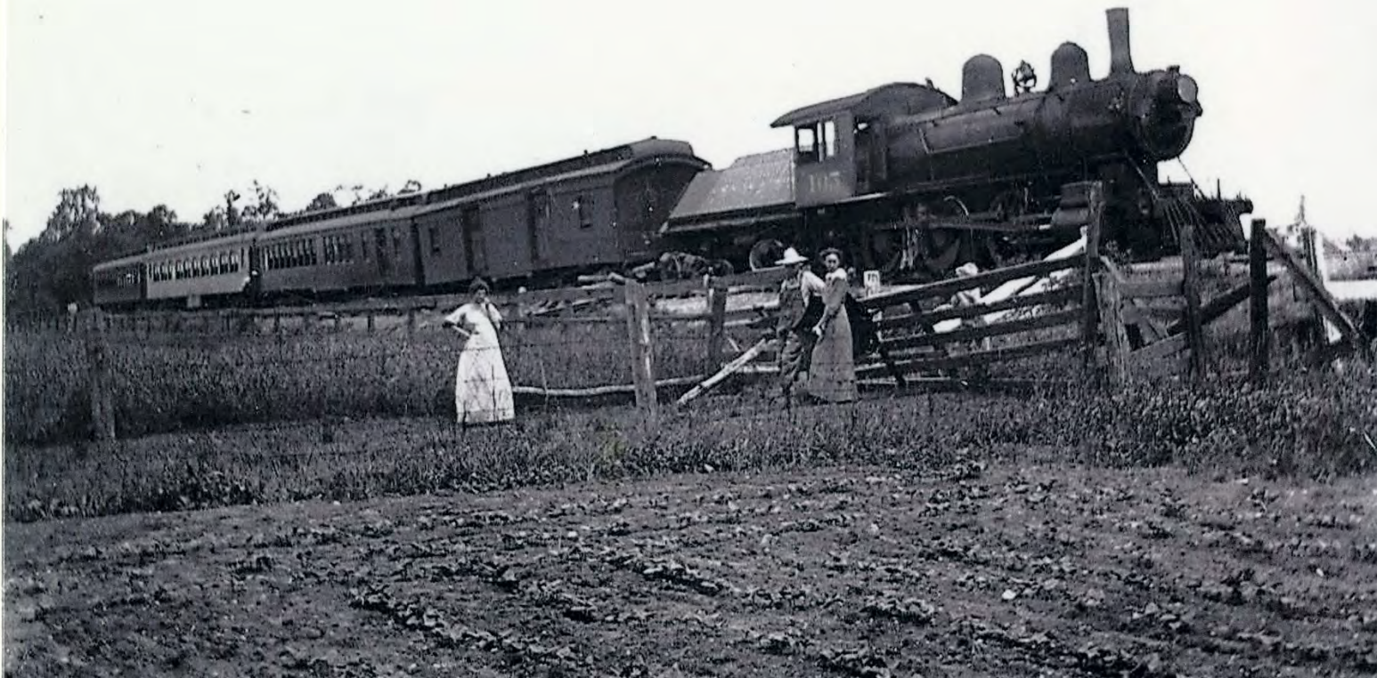
Photo #1: The photographer was early at the scene as only a few persons are about in the farm lane. This view is from the west side of the tracks looking northeast. The Salt River Cemetery would be to the left several hundred yards. The four car train consists of the baggage car, combination mail & passenger car and two regular passenger cars.
