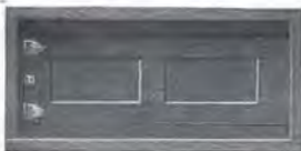
Panel in Ceiling—looking up
