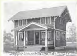
Front View of Georgia No. 1
