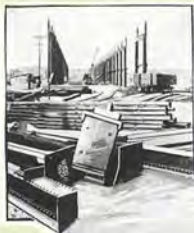
Redi-Cut System of Construction.
