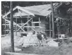
Progress of Work Seventh Day
