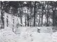
Starting Construction First Day
