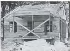
Frame Work Up on Third Day
