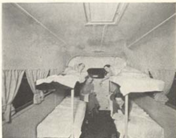
Four Berths Made Up. Note Spacious Floor Space
