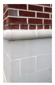
Rough cut limestone, chamfered concrete cap, new brick and concrete frame application.
