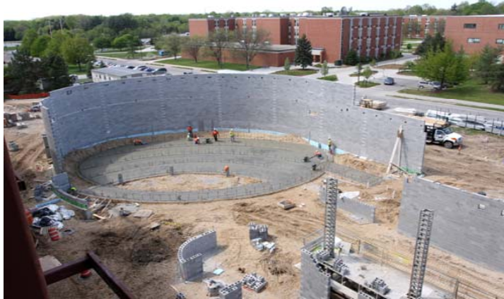
Laying the foundation
